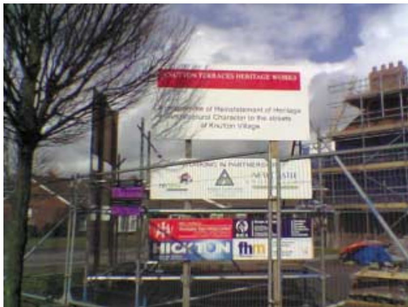
Picture Above: Heritage Work continues at Knutton Village
