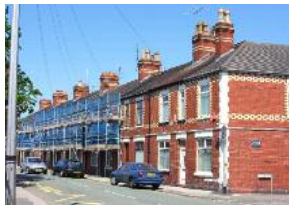
2008 Work in Progress at Lawson Terrace, Knutton
