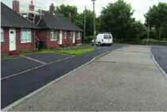
Stanton Close after the bungalows have had individual driveways created.
